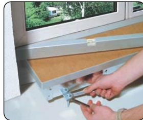
Horizontal fitting with adjusting screws
