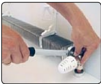
Connecting supply pipe
