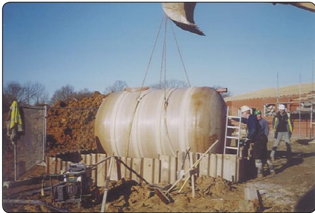
Installation of 12,000 litre rainwater storage tank at Queenswell Infants School, London
