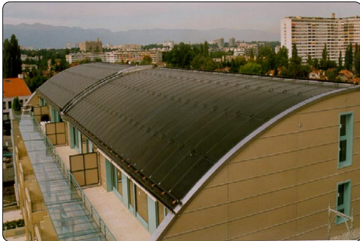
The ES Solar Roof has been used here to roof an apartment block in Switzerland showing how it readily follows a curved profile.
