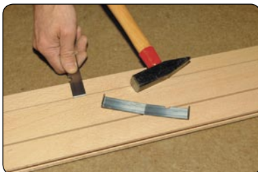
Use of the optional clip system minimises the need for glues (refer to information sheet WF2)
